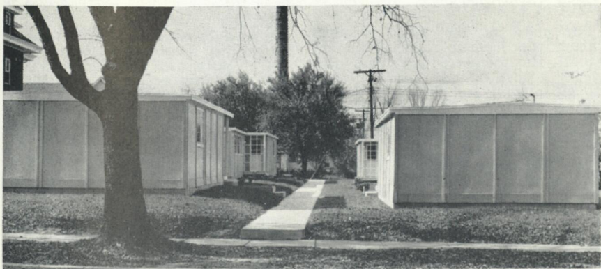
Pictured are four faculty annexes which have provided additional classroom and laboratory space, and faculty offices.
