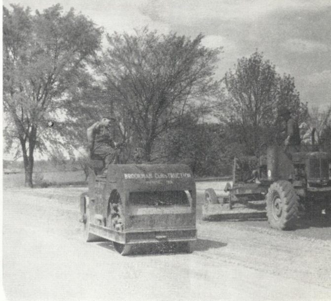
Laying the base for the asphalt recreation area
