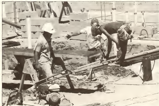
Construction of the new Samuel Morris Hall began in the summer of 1997 and is expected to be completed in the spring of 1998.
