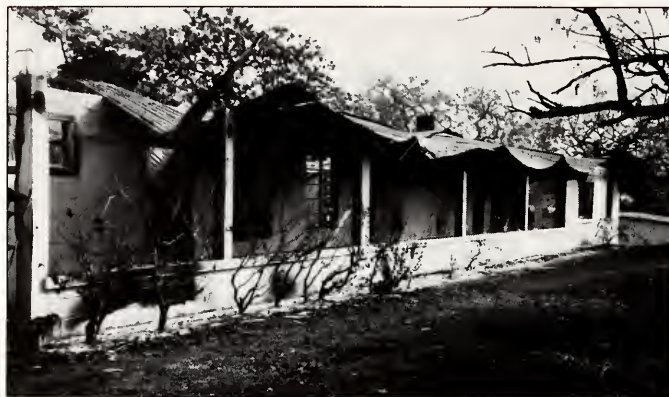
The “Teacher's House” after the fire.
